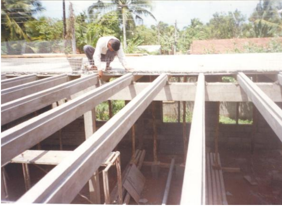
Laying of prestressed purlins
